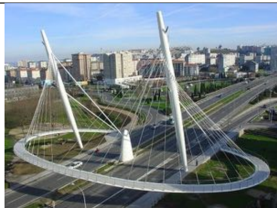
Cable stayed bridge with weight supported in optimal area - Pasarela Atirantada "La Rosa"
