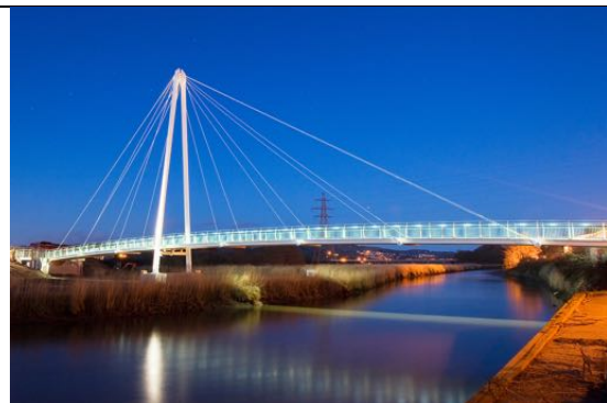
Cable stayed bridge with weight supported in optimal area - Newton Abbot
